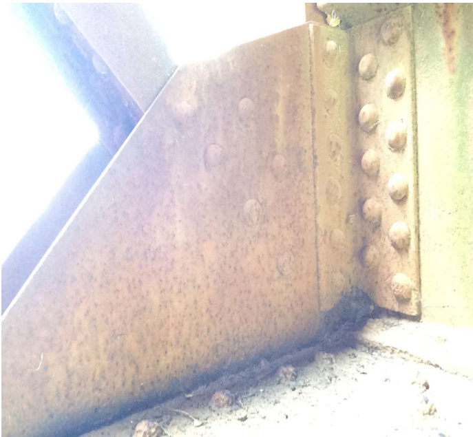
PHOTO 7 Description L4 Left Interior gusset at the Floor beam connection.
