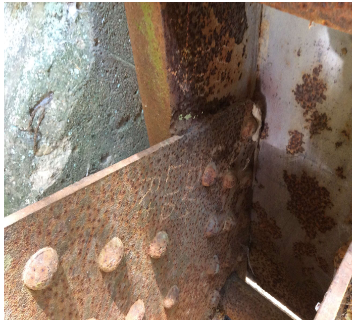
PHOTO 5 Description L10. Right. Hole rusted through the interior channel of the end post.
