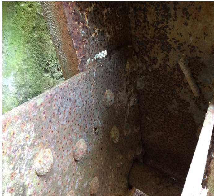
PHOTO 1 Description L0. Left hole rusted through the interior end post at the gusset connection
