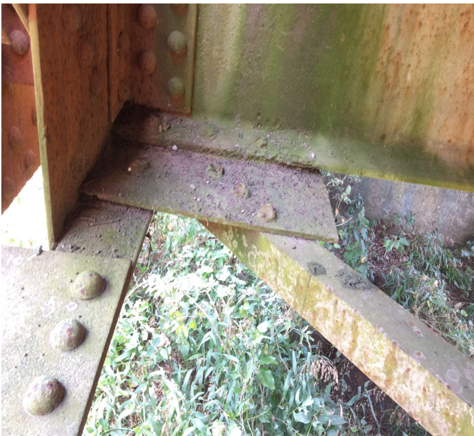
PHOTO 4 Description L2. Right. Lower lateral gusset connection
