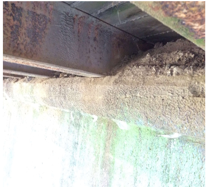
PHOTO 2 Description Bent 1 cap. Dirt on stringers.
