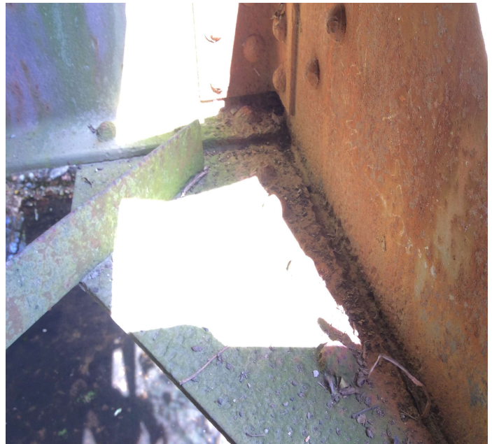
PHOTO 9 Description L4. Right. Interior. Lower gusset connection
