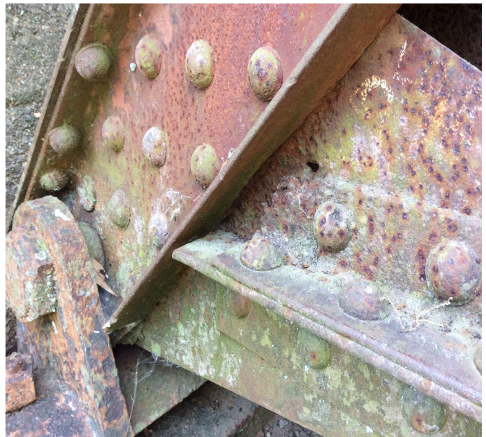
PHOTO 6 Description L0. Right. Exterior connection plate with 1/4" hole.
