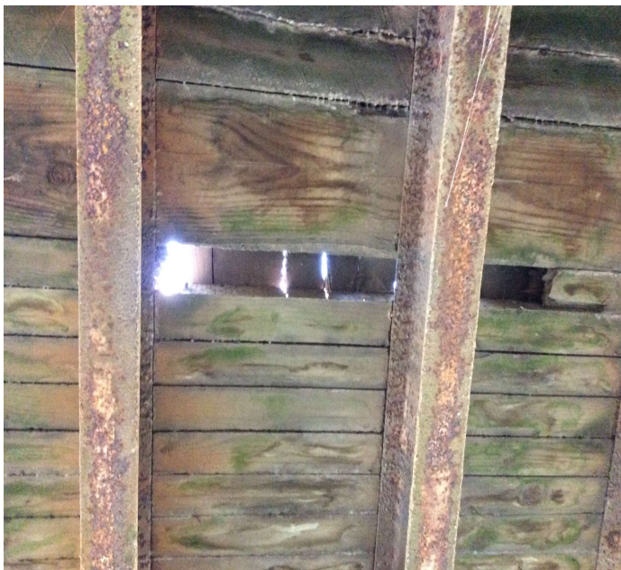
PHOTO 3 Description Deck soffit. Bay 1. Right wheel path.
