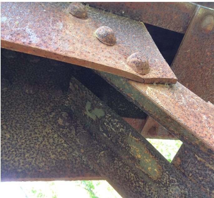
PHOTO 1 Description U5-L6 at U5. Right. 1/8" crack with out of plane bending. No change.
