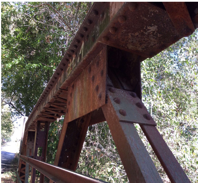
PHOTO 3 Description U7 connection plate.
